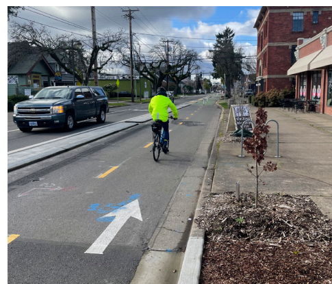
Two way separated bike lane, bicyclists and vehicles are separated by a curbed median
