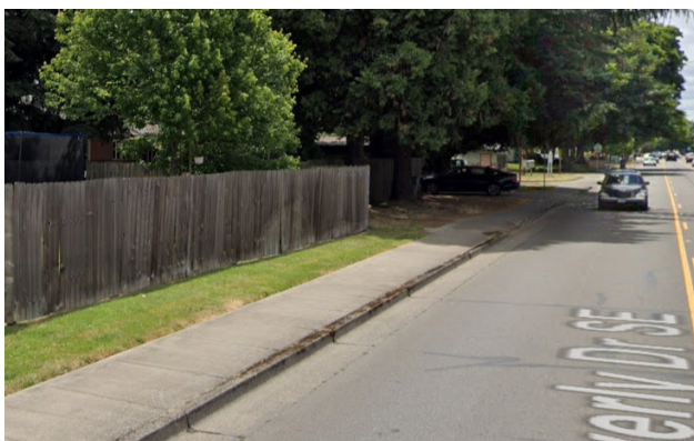
A curb tight sidewalk along Waverly Drive in Albany. Photo from Google Maps Street View.
