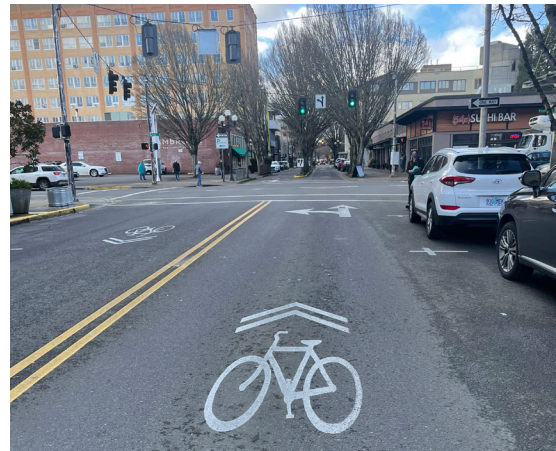
Shared lane with sharrow marking
