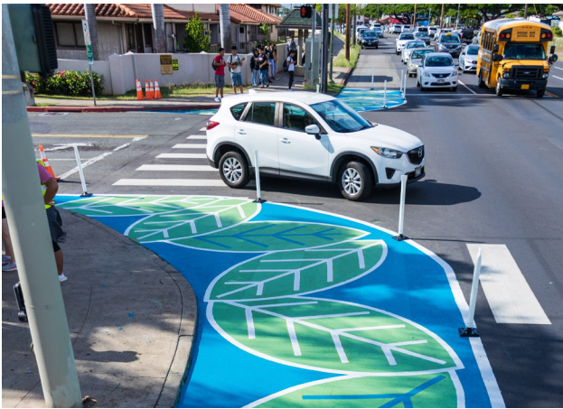
Painted curb extension in Honolulu, Hawaii. Image from Ulupono Initiative.
