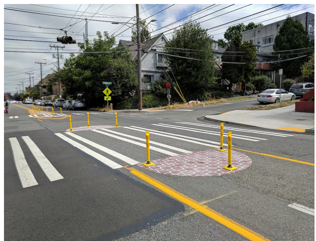
Temporary crossing island. Image from Seattle Right-of-Way Improvements Manual.
